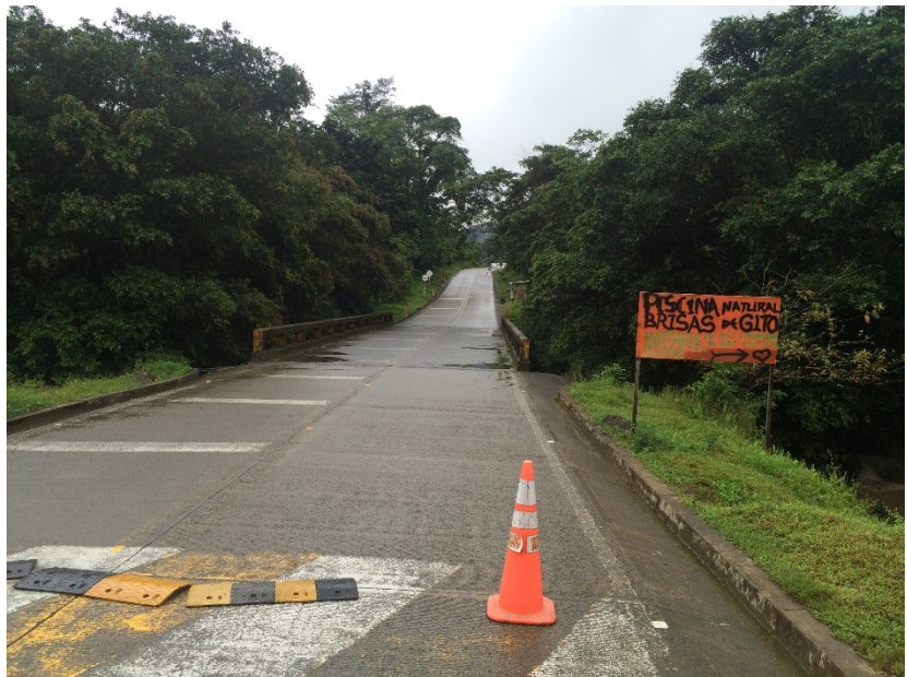
Bridge at Gito, park at the military checkpoint on the right and walk upstream
